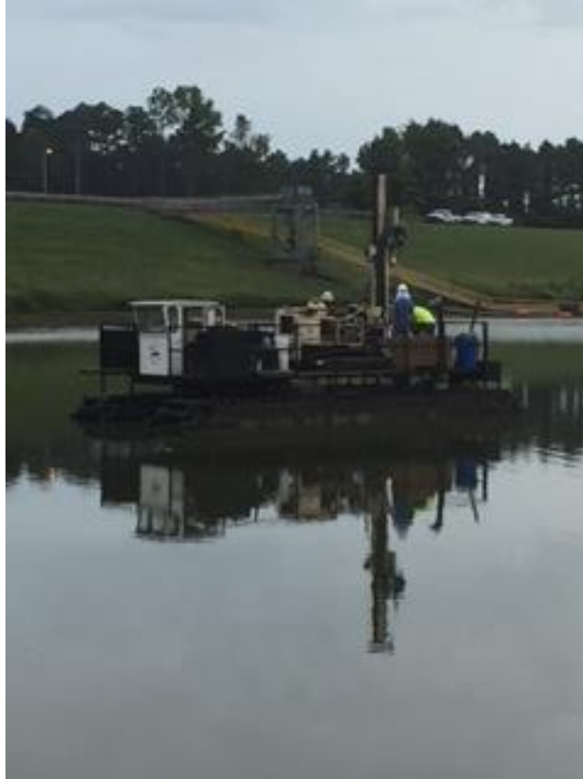
PHOTOGRAPH 1 Bottom Ash Pond - Typical Geotechnical Drilling Rig Setup.
