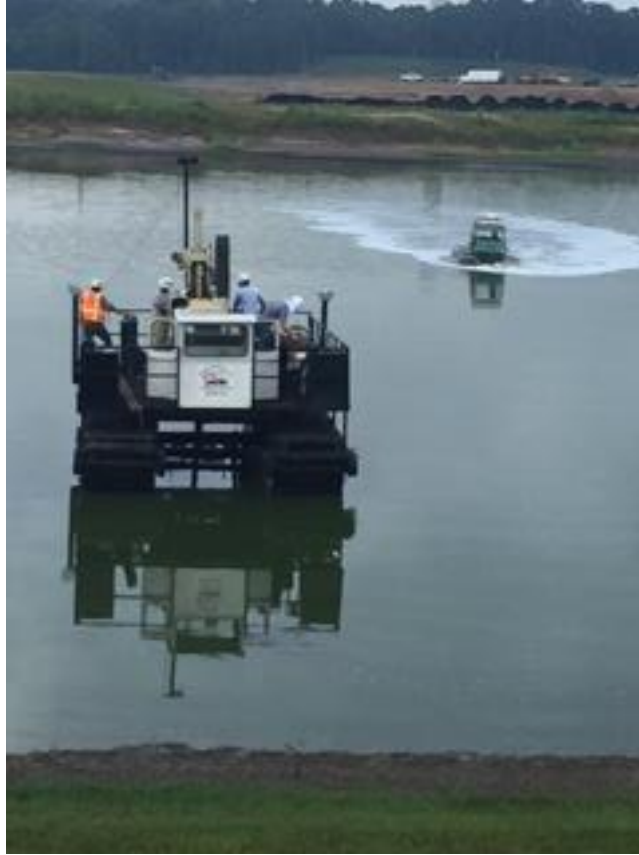
PHOTOGRAPH 1 Fly Ash Pond - Typical Geotechnical Drilling Rig Setup.
