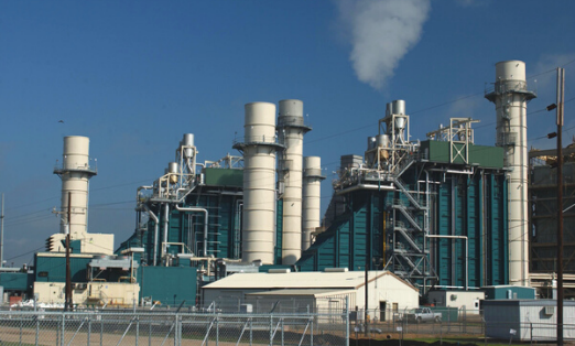
Coughlin Power Station
