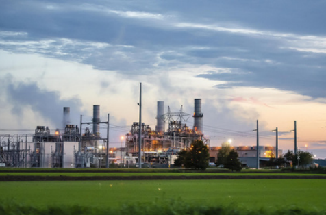
Acadia Power Station
