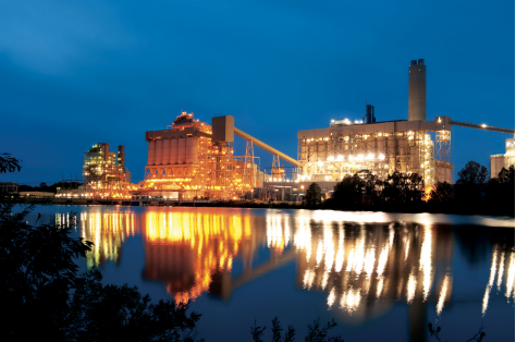
Brame Energy Center
