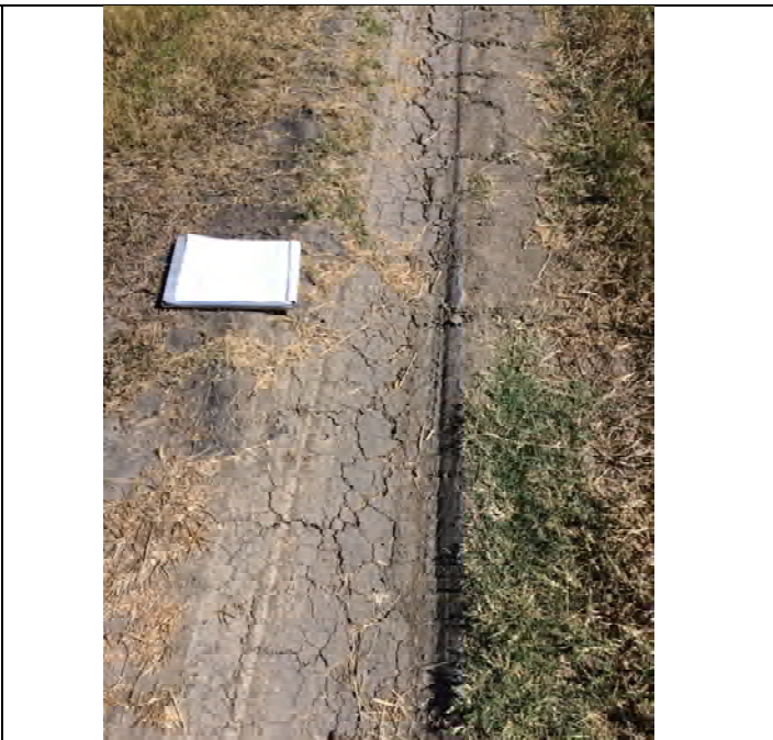
Photo No: 7 Picture Direction: E Photo No: 8 Picture Direction: E Description: SW corner of Fly Ash Basin looking along south levee Description: Tension cracks in road surface at a slough in SW corner of Fly Ash Basin.
