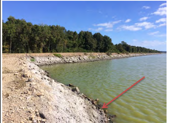
Photo No: 5 Picture Direction: W Photo No: 6 Picture Direction: W Description: Example of erosion protection undercut along north Fly Ash Basin levee. Description: NW corner of Fly Ash Basin. Note coloration of rocks indicating the high water mark.
