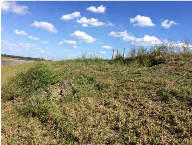
Photo No: 13 Picture Direction: W
