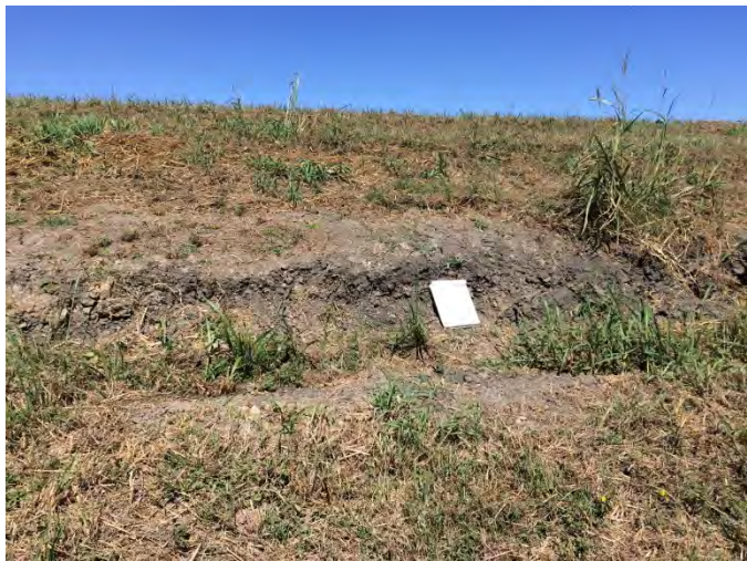
Photo No: 9 Picture Direction: N Description: Slope escarpment below tension cracked section along south levee of FAB
