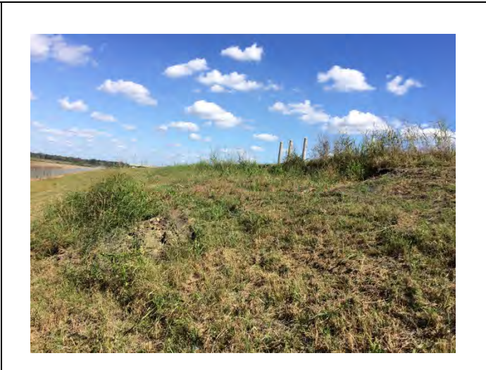
Photo No: 12 Picture Direction: S Description: Slough and bulge of Bottom Ash Berm near northeast corner.
