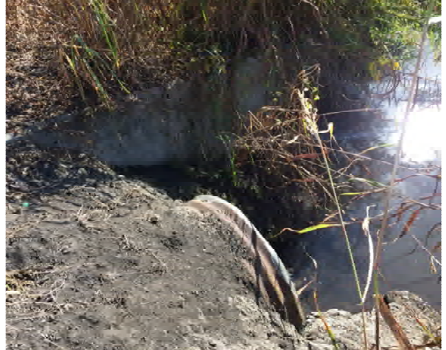
Photo No: 14 Picture Direction: W
