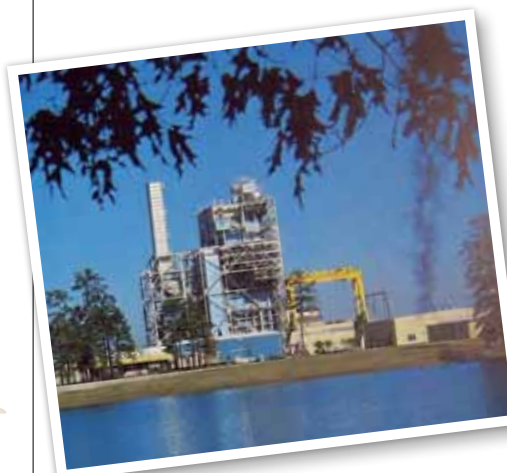
The Rodemacher Power Station, built on Rodemacher Lake, opened in 1975.
