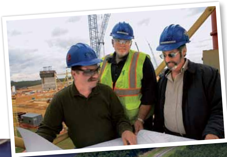
LEFT: Clark Bordelon (from left), David Lee, and Lenny Kliebert review plans for Rodemacher Unit 3 with circulating fluidized-bed “clean coal” technology. Construction began in 2006.
