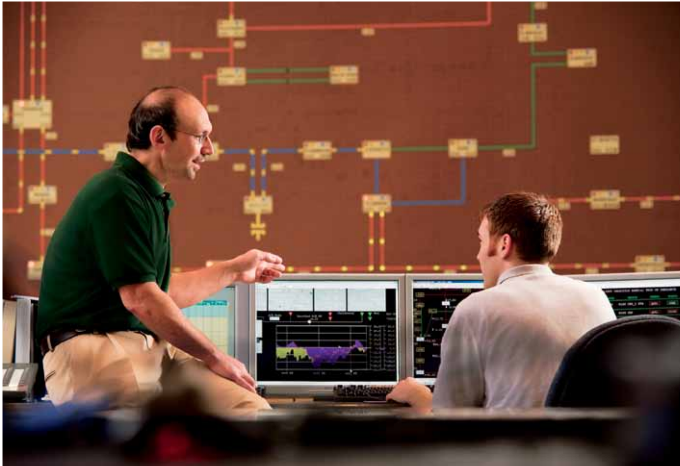
Upgrading transmission was a priority for Cleco in the mid-2000s. Here, Terry Whitmore (left) and Christopher Thibodeaux discuss expansion plans in the Coughlin Transmission Operations Control center.
