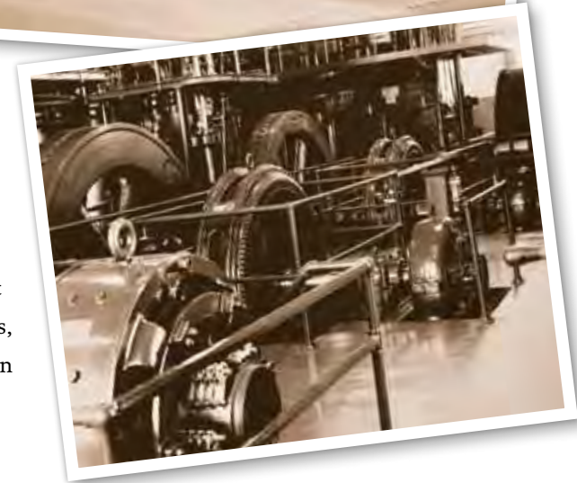
ABOVE: Upgrading this rundown ice plant was just one of the challenges Cleco acquired in the Gulf Public Service merger.
