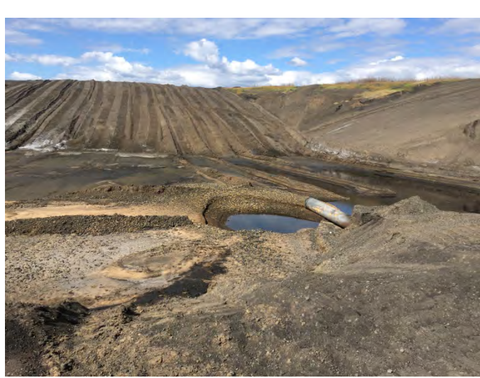
Photo No: 26 Picture Direction: N Description: Southeast corner of the Bottom Ash Unit discharge slurry discharge point into the Bottom Ash Unit
